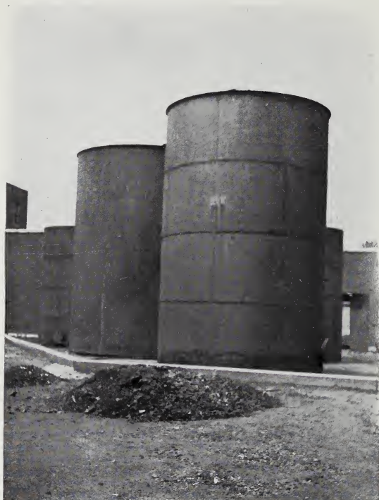
FIG. 53.—Turpentine Tanks. Louisville Varnish Co.
